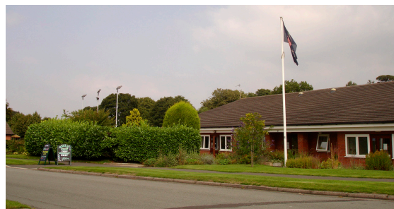
Delamere Park Clubhouse
